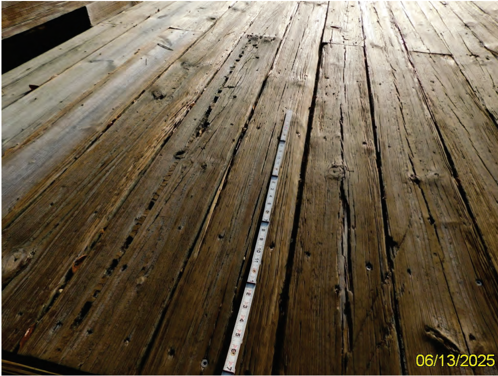
Photo 6 – Timber Deck (Wearing Surface)
