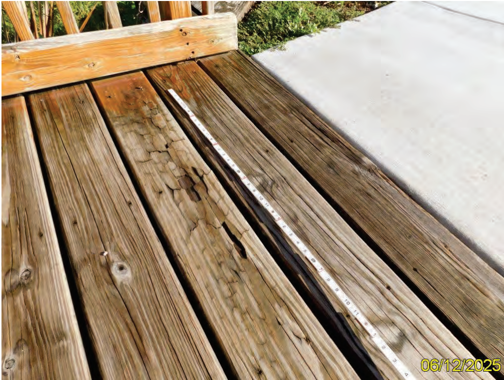
Photo 4 – Timber Deck (Wearing Surface)
