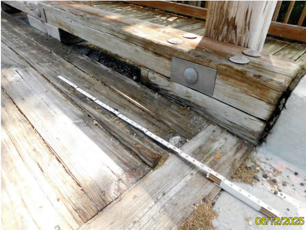
Photo 5 – Timber Deck (Wearing Surface)
